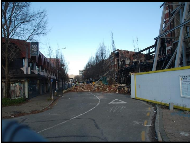
Photo 1: Blocked City Street and Unusable Buildings in the CBD - July 2013
