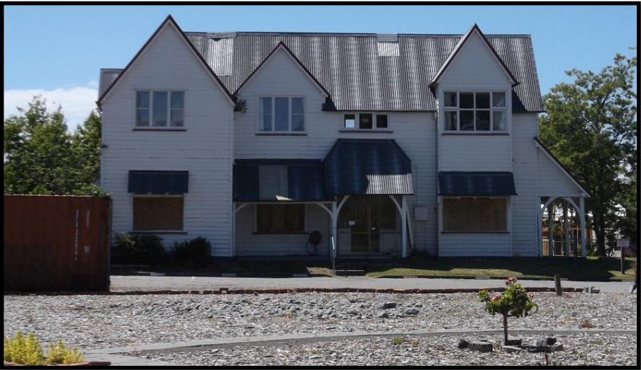
Photo 4: Damaged Home on the Outskirts of the CBD with Lot of Demolished Home in Foreground - November 2014
