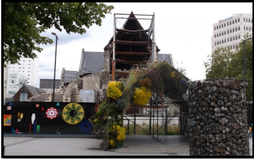
Photo 7: Christchurch Cathedral Damages - November 2014
